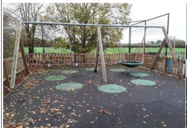
**Finding:** Swings of this design should have a secondary safety device fitted to prevent collapse of the seat in the event of a joint failure to meet the requirements of BS EN 1176 Part 2
