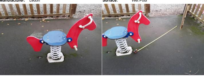
**Finding:** The gate forms a hard object within the impact area of the equipment when in the open position
