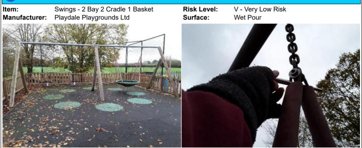
**Finding:** The chain openings are in excess of the 8.6mm as **Action:** Monitor - No remedial work recommended recommended by BS EN 1176
